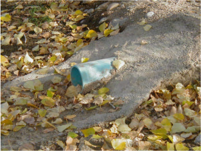
Unscreened storage tank overflow
