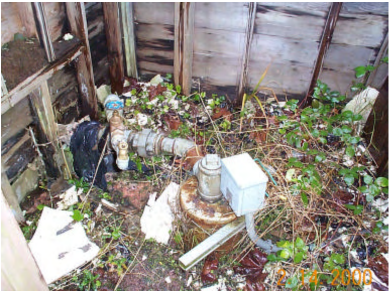
Poor housekeeping of the well house
