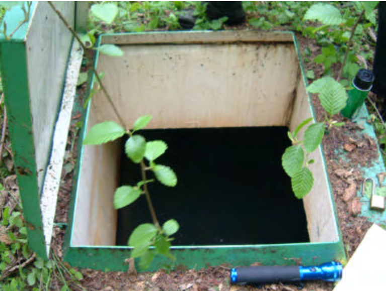
Unsealed -storage hatch cover
