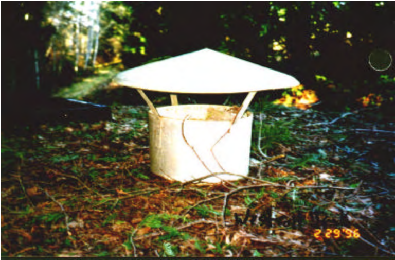
Unscreened storage tank vent
