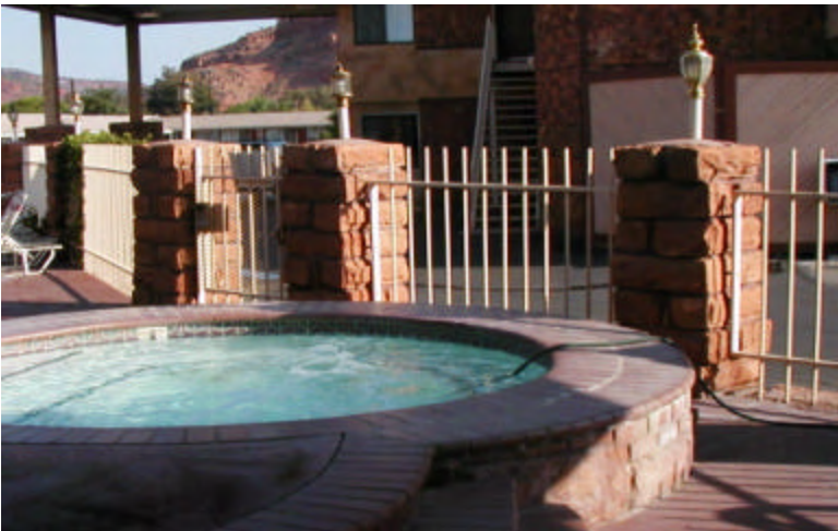
Fill hose with no air gap, creating a cross connection hazard
